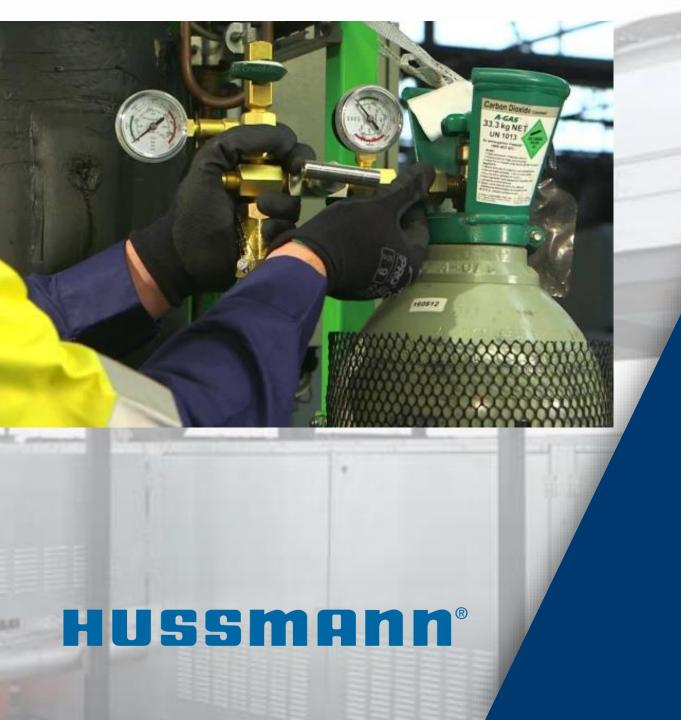
Due to its physical properties, CO<sub>2</sub> charging must be done in 2 stages: First with gas, and then with liquid
